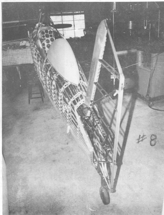
Not realizing at the time that it put the bottom rear of the tank past the cross piece of tubing on top of frame. By that time the rear of tank was welded in place. The front panel was held in place with duct tape, not yet riveted. (Lucky Me)
